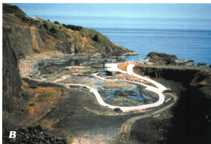
Figure 27. Quarry Cove, Yaquina Head Outstanding Natural Area, Newport, Oreg. Photographs courtesy of Bureau of Land Management, Salem District. A, View of worked-out quarry. B, Transformed cove at low tide; quarried below sea level with site open to the ocean.
