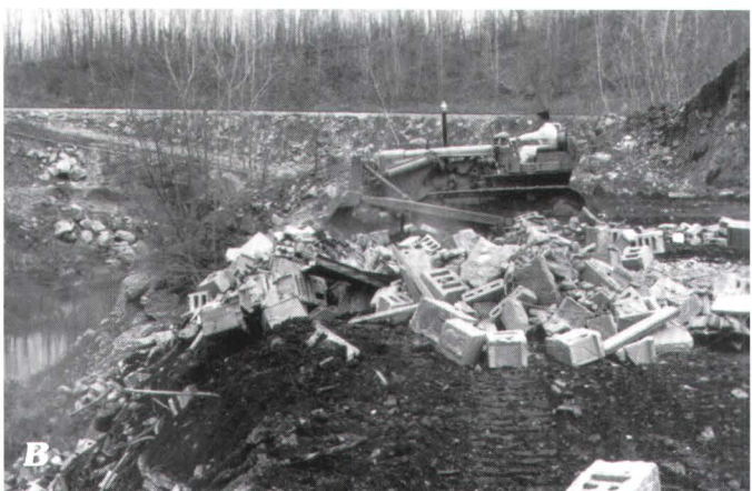
Figure 13. Quarry at Weldon Spring, Mo. Photographs courtesy of Morrison Knudsen Corporation, St. Charles, Mo. A, B , The visual effect of dumping operations from 1940's to 1960's. Waste types included TNT/DNT, thorium, radium, and uranium. C , Excavated quarry basin.
